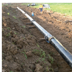
TT PE pipe train ready to be pulled by horizontal directional drilling
